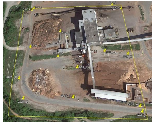
Figure 5: Ground Control Point Layout
